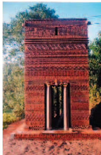
Turmbau in Bhaktapur
