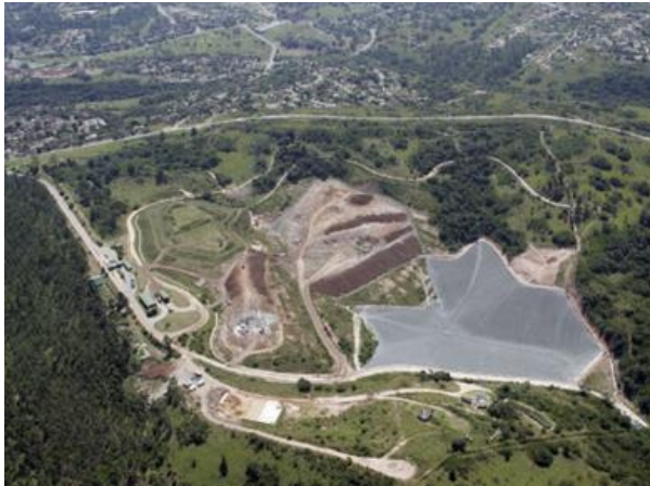
Figure 40: Aerial View of the Mariannhill Landfill Conservancy Plant. Source: (Cauchois, 2014, p. 2)
